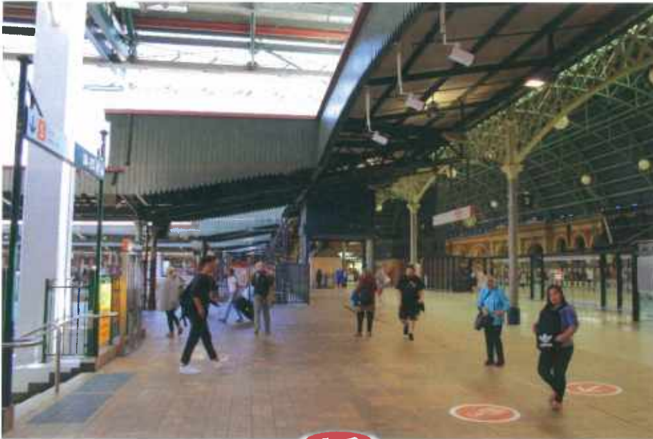
Figure 1: Platform access area between the Main Concourse and Intercity Platforms showing bridging structure at the northern end of Platforms 8/9.
