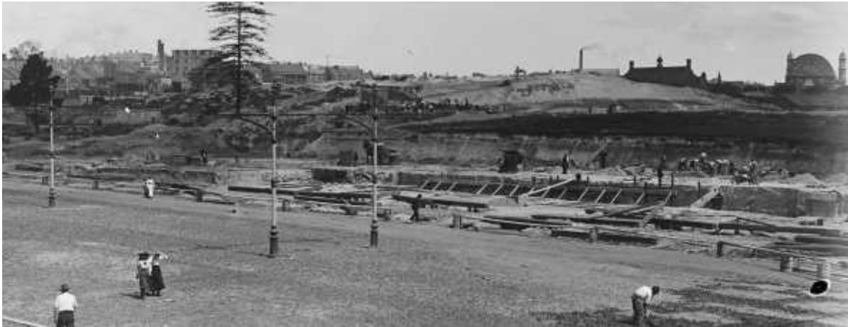
**Figure 6: Excavation of the sand ridge for the new station and construction of Eddy Avenue**
